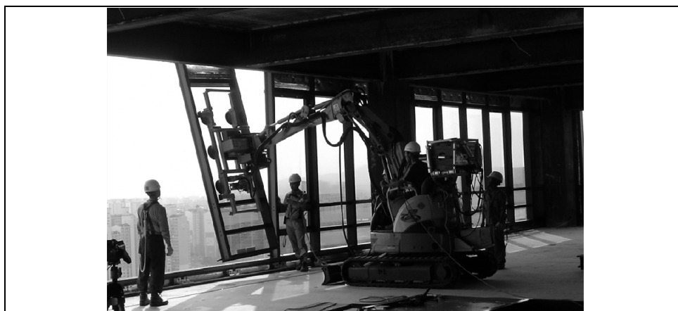
Fig. 2. An ASCI (Automation System for Curtain-wall Installation)
